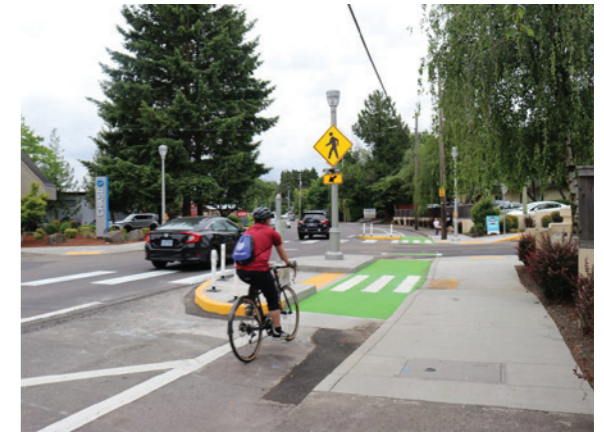
Protected bike lane and highlighted pedestrian crossing at intersection in Portland, Oregon
