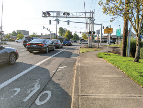
Intersection at Gable Road and Highway 30.
