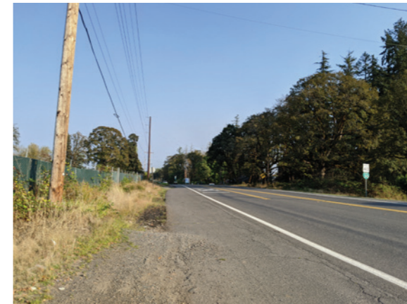
A majority of Gable Road and Old Portland Road do not have sidewalk infrastructure
