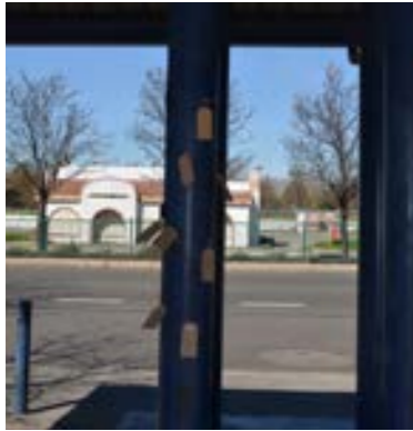
The column, with all the tags put in place
