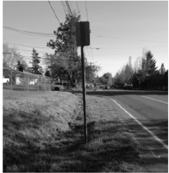
View of southwest corner of project site looking towards the intersection of SW 72nd Avenue and SW Baylor Street
