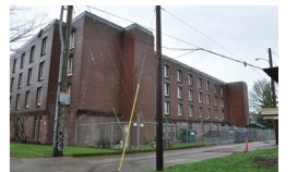
Building facing the Alley
