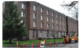
Building facing Jarrett St
