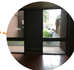
Existing East Lobby
