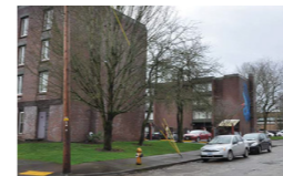
Building facing Kerby Ave
