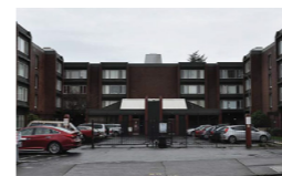
Building facing Kerby Ave
