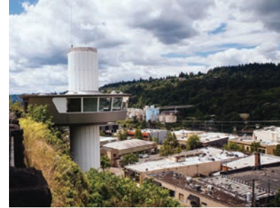
Oregon City Municipal Elevator
